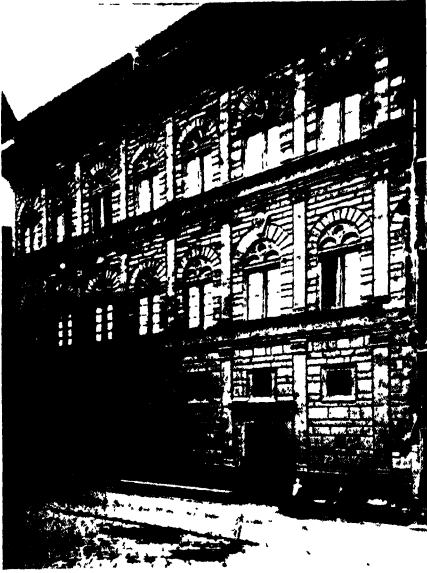
159. Palazzo Rucellai, Florence Designed by ALBERTI about 1460
